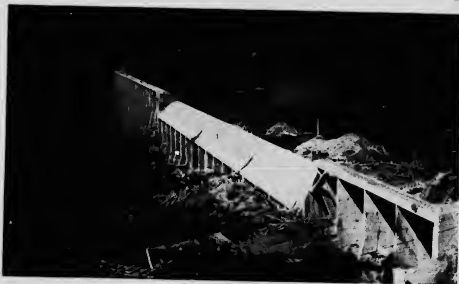
Vancouver Island Power Company Limited. East end of Jordan River Dam showing spillway.
